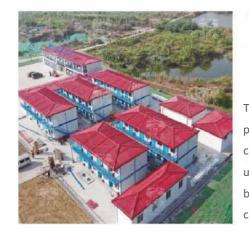
The K house is a kind of light steel as the skeleton, with the sandwich panel as the enclosure material, with the standard modulus series are combined in space, and the color steel prefabricated house components use bolts connection, the standard size of the prefabricated house base box is 3.64\*6.16, Custom sizes available upon request. It is widely used in construction sites, warehouses, etc., exported to Southeast Asia, Africa.
