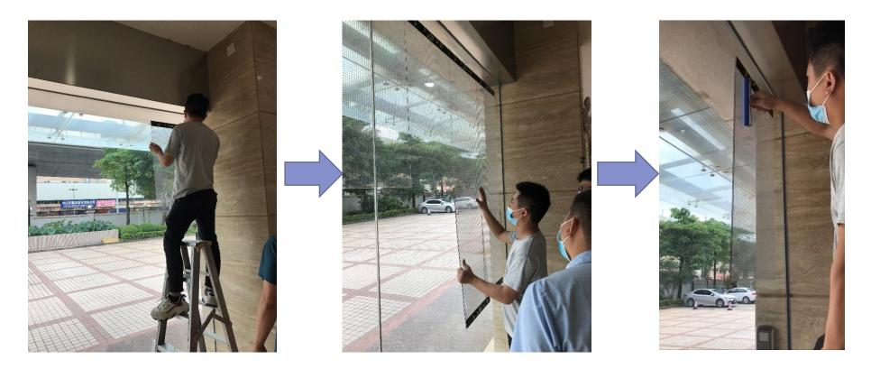
The first step is to wipe clean the glass to be installed The second step is to apply the product directly on the glass The third step, use the scroll wheel to scroll on the product
