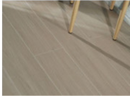
Single chip specifications: 1220 x 202 x 12mm MDF: 780/m 3
